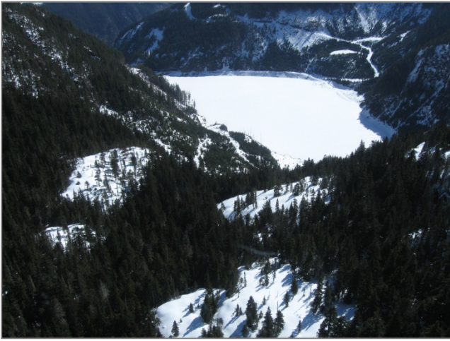
Arrowsmith Lake Reservoir (April 2009) - looking north
