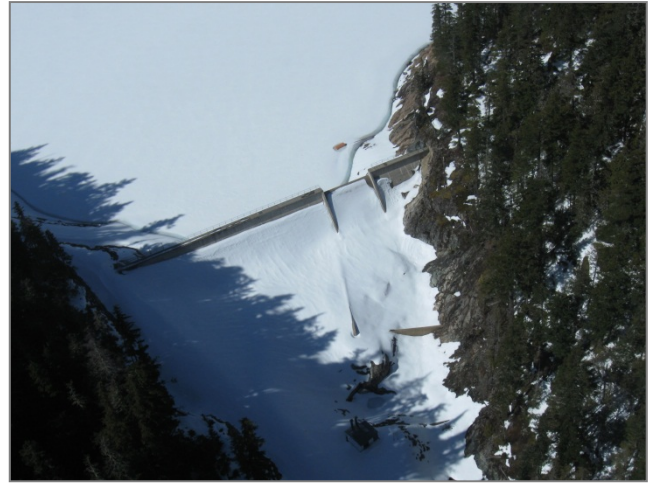
Arrowsmith Dam (April 2009)
