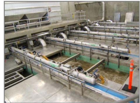
Water Treatment Facility – City of Kamloops
