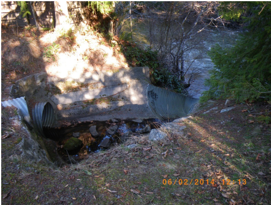
Figure 13: Looking northeast at concrete culvert on west shore of Englishman River in Segment 10.
