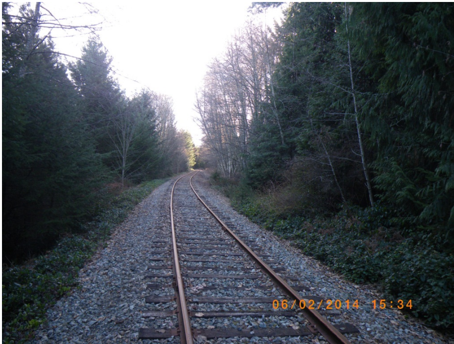
Photograph 3: Looking southeast along E&N Railway right-of-way in Segment 2.
