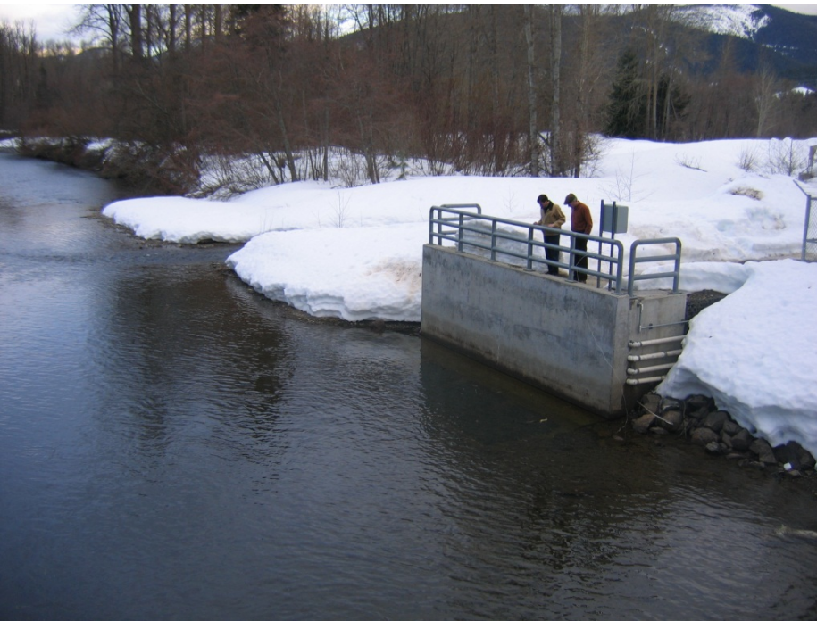
Figure 9: Looking towards proposed surface intake at Segment 7.
