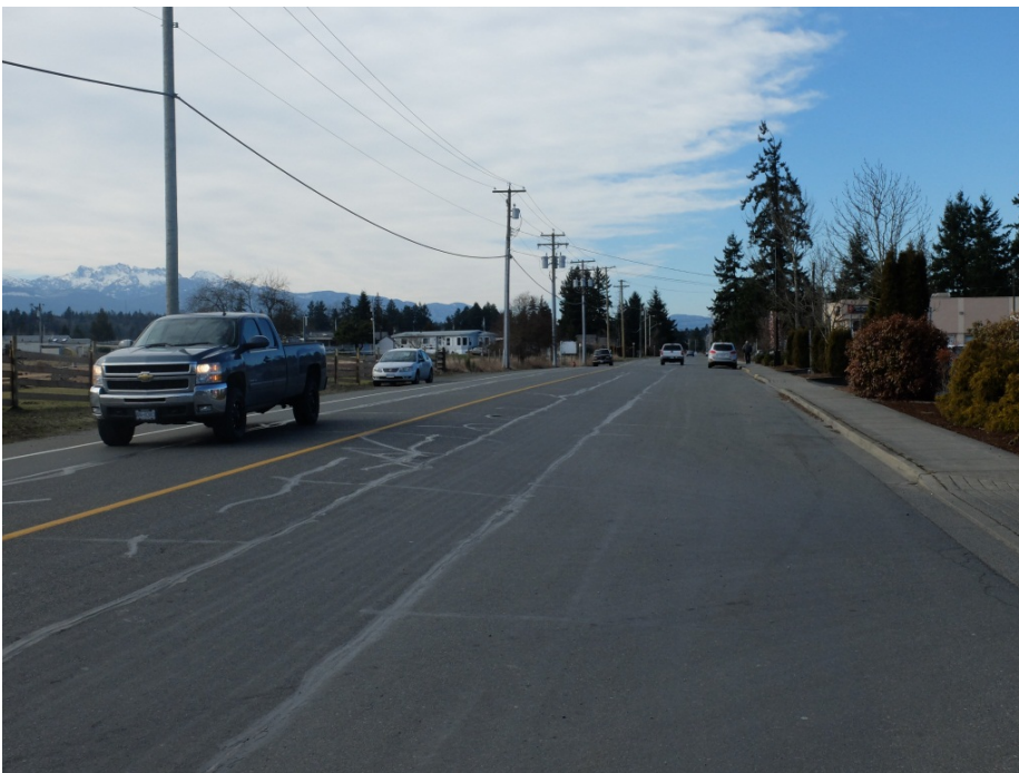
Figure 8: Looking west along Stanford Avenue in Segment 6.
