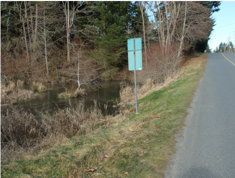
Figure 7: Looking north along west side of Martindale Road in Segment 5.
