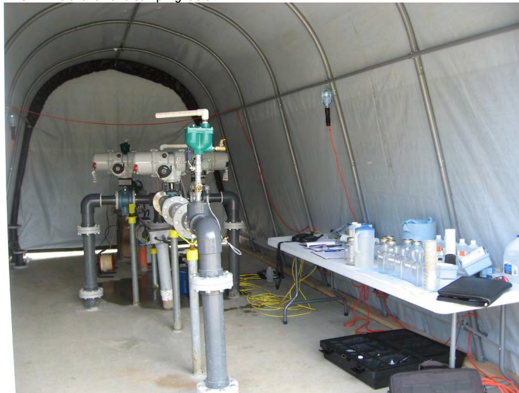
ASR-1 installation and sampling table
