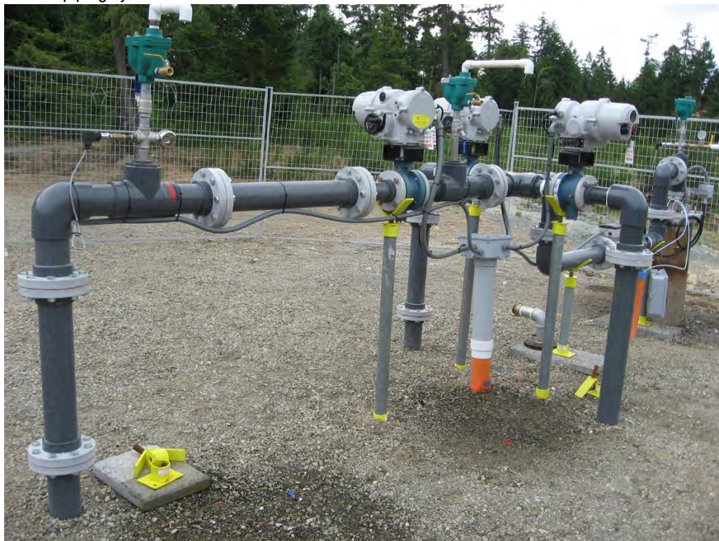
ASR-1 piping system
