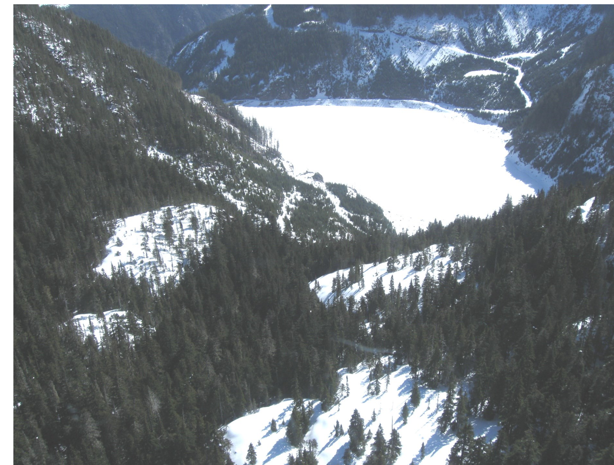
Arrowsmith Lake Reservoir (April 2009) - looking north
