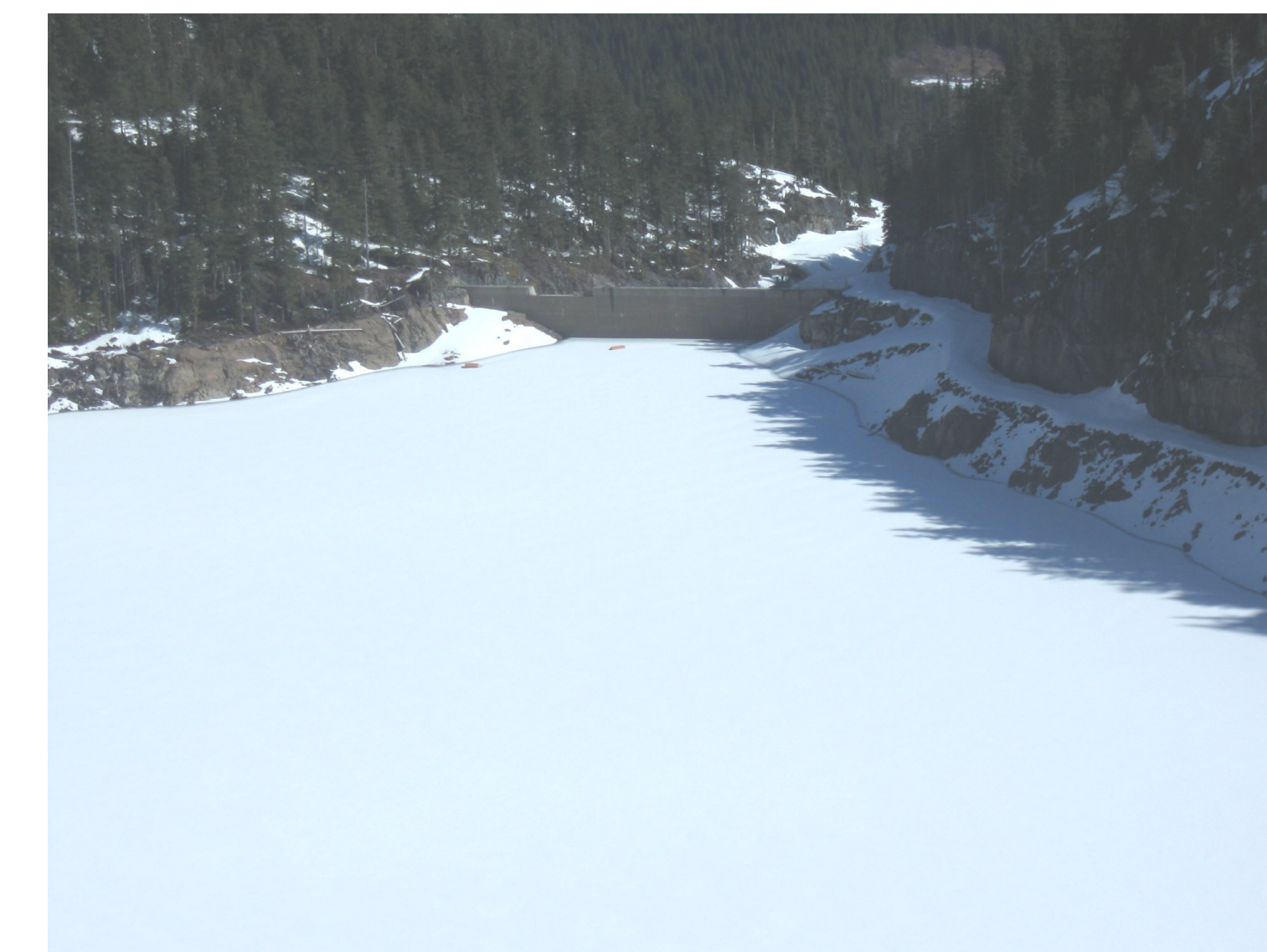
Arrowsmith Lake Reservoir (April 2009) - looking north
