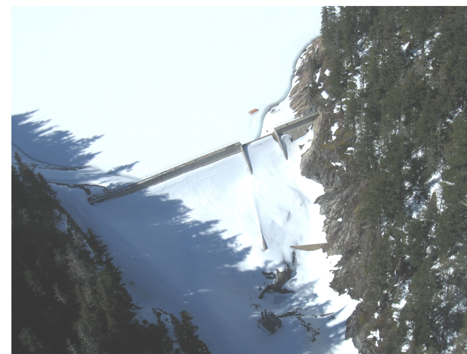
Arrowsmith Dam (April 2009)
