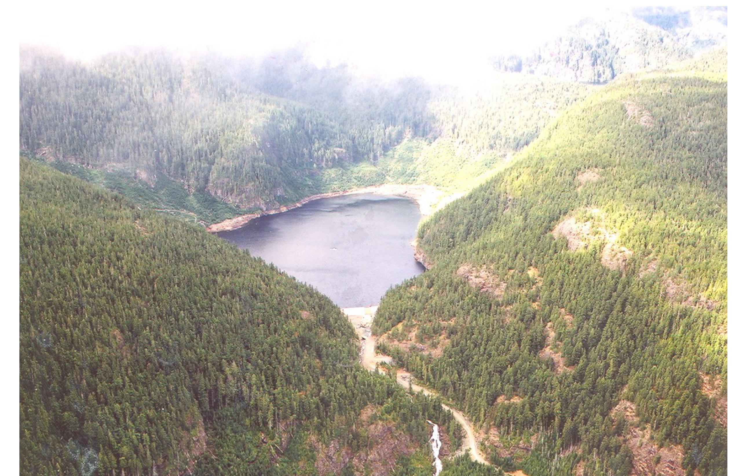
Arrowsmith Lake Reservoir in Operation (Summer 2002)
