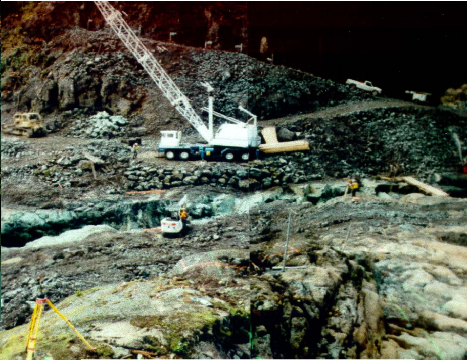
Arrowsmith Lake Dam Construction - 1998
