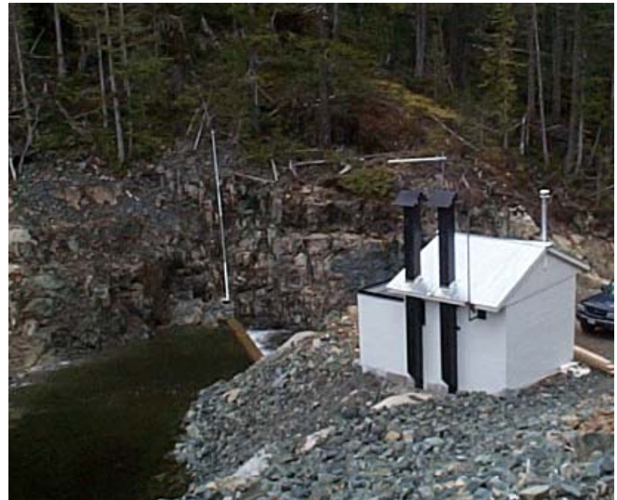
Arrowsmith Dam – Control Station
