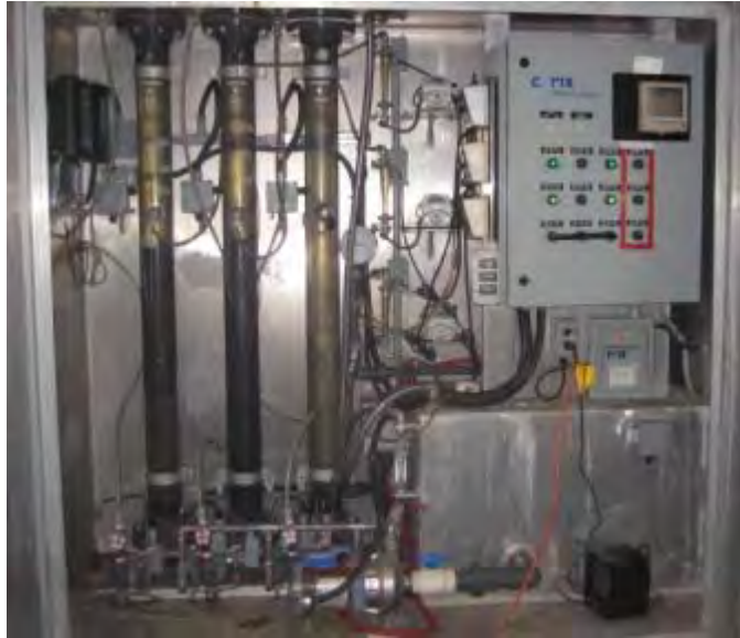
Figure 3-4 - Conventional Treatment Pilot – Filter Columns
